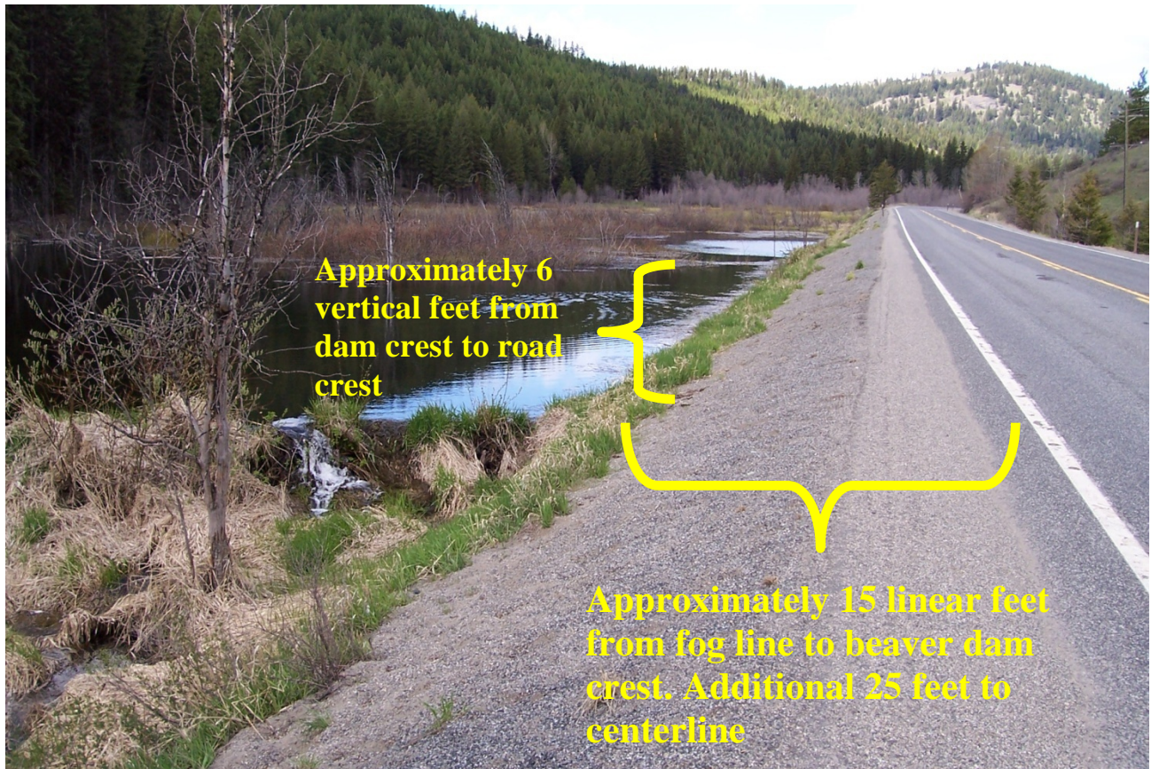
Figure 4. In this photo, the roadway is directly adjacent to a beaver dam complex on Granite Creek near Republic, Washington. The distance from fog line to the edge of the water measures approximately 15 horizontal feet, and the distance from dam crest to the top of the roadway measures approximately 6 vertical feet. Photo by Brian Walker.
