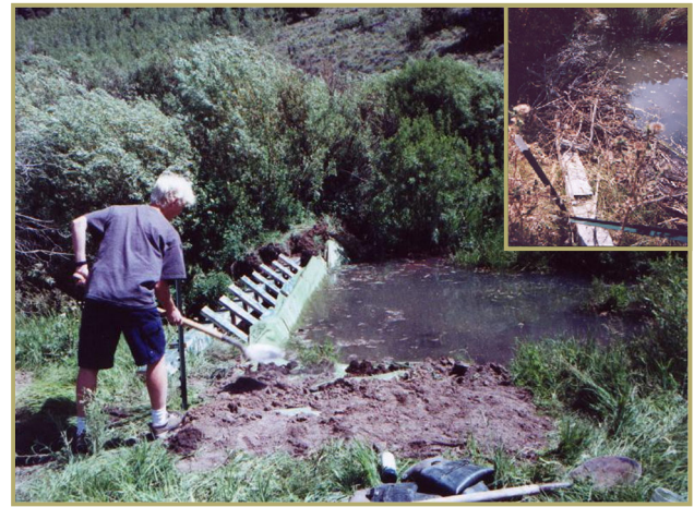
Fig. 4 Example of reinforced beaver dam in southwestern Idaho. Five beavers were translocated and released at this site, which resulted in a new dam built on top of the instream structure (inset) and additional dams built upstream of the release site
