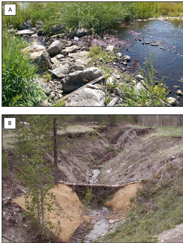
Fig. 3 Examples of two types of artificial structures (designed to mimic some of the effects of beaver dams) used in stream restoration projects. a) A rock structure dam installed by a private landowner in eastern Oregon and referred to as an “artificial beaver dam.” b) A wood structure installed by a private organization in western Montana and referred to as a low-profile wooden dam
