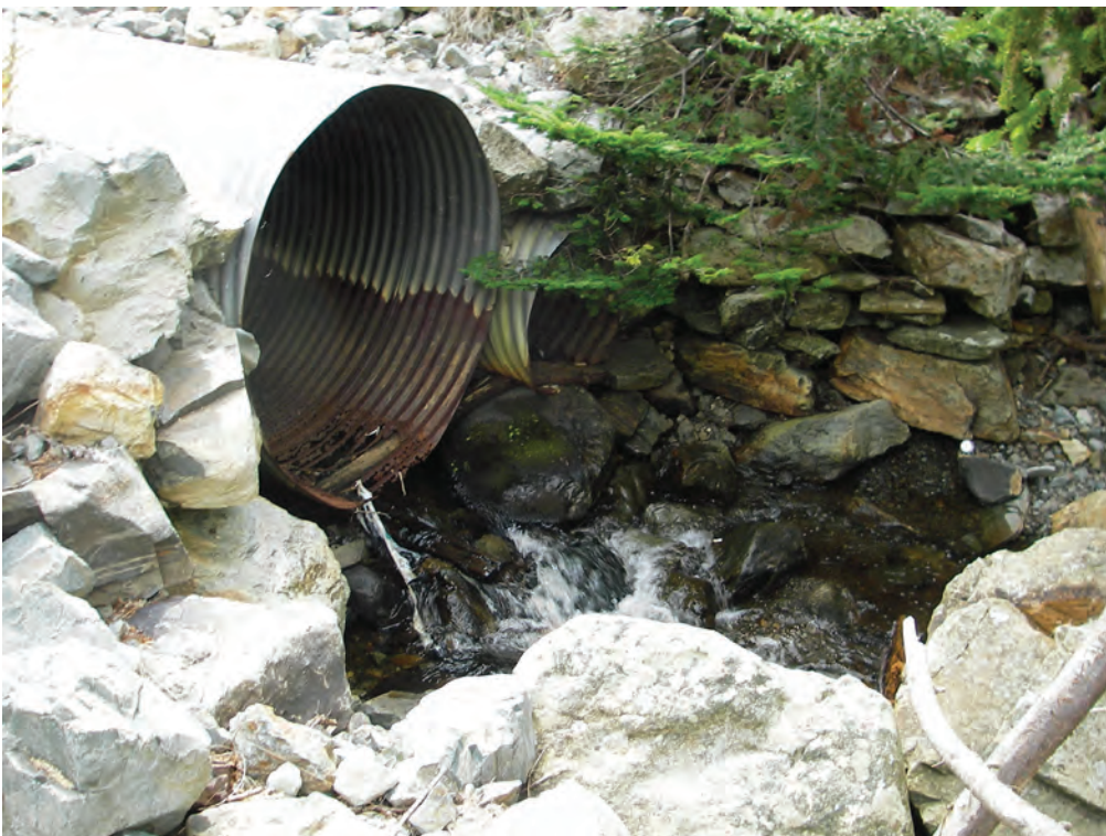
(b) Blocked culvert outflow
