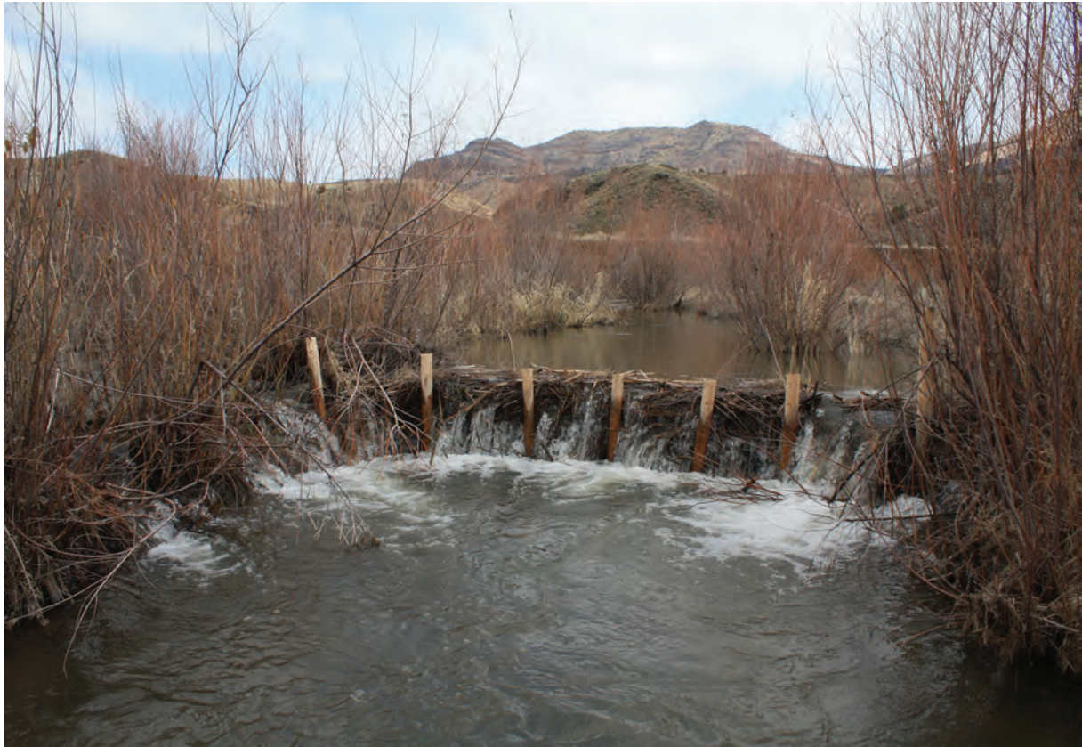
Figure 3 Beaver Dams Support (BDS) structure designed to assist North American beaver dam construction in the incised Bridge Creek, Oregon, United States (photograph provided by M. Pollock).
